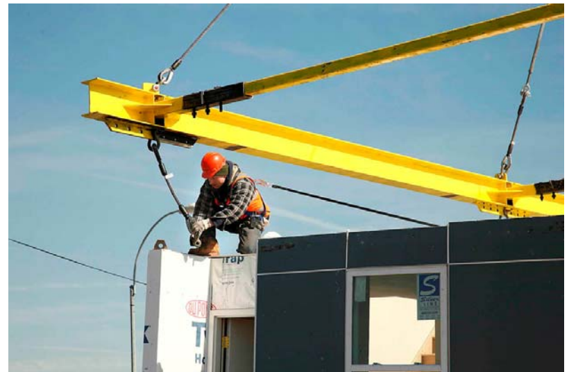
HPD Contractors hard at work
